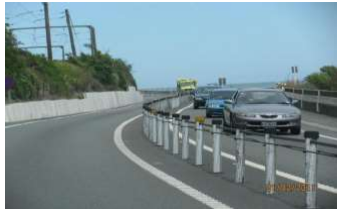
Fig.3: Flexible cable barriers
