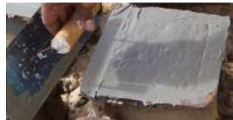
Fig.2: placing and finishing.
